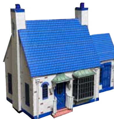
Gas Station, Pure Oil Standard "Cottage" (1920) Cape Charles, Virginia
