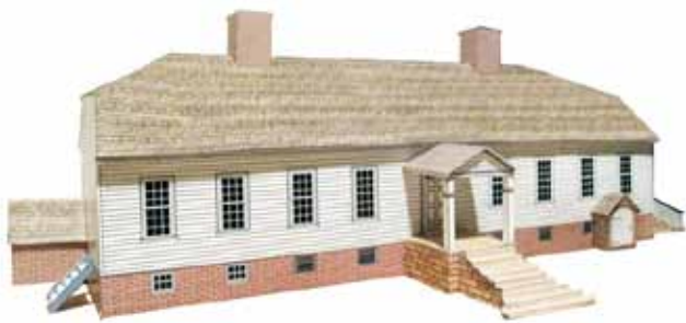
Scotchtown (1720) Hanover County, Virginia * A Preservation Virginia Historic Site
