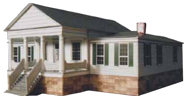
Craik-Patton House (1834) Charleston, West Virginia *
